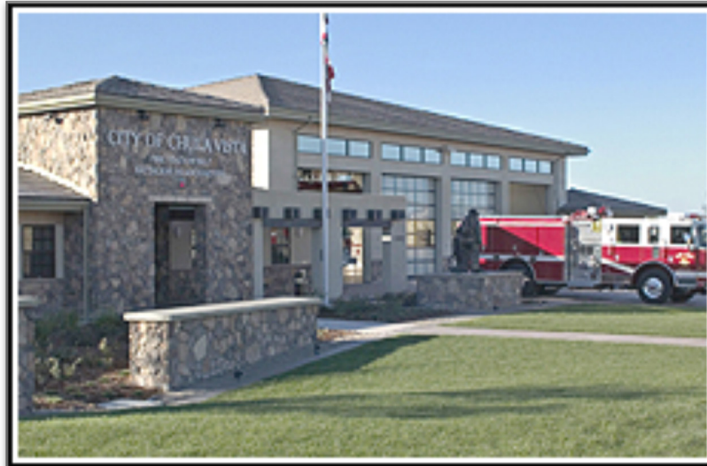
Fire Station in Otay Ranch
