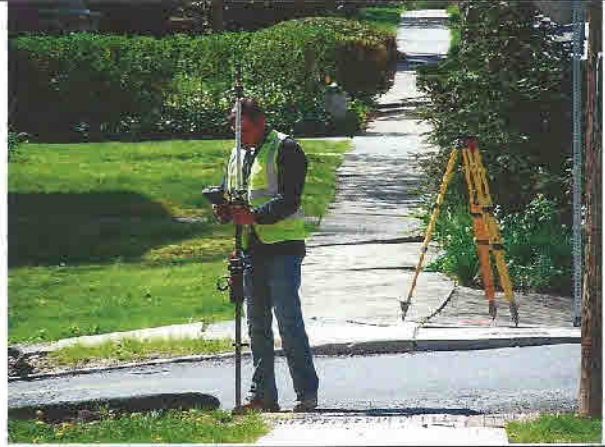
Careful Excavation by COE Public Works Department
