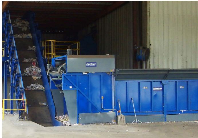
North Augusta Material Recovery Facility
