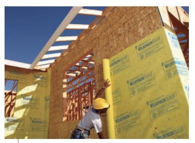
Every house needs a WRB. A properly detailed waterresistive barrier such as asphalt felt paper or plastic housewrap prevents water that gets behind the siding from doing any damage. It's important to tape housewrap seams and overlap them "shingle style" so they shed water.
