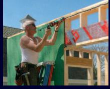
Sheathing air barrier. Panel sheathing makes an excellent air barrier. Seams should be sealed with long-lasting, high-stick tape, and holes should be plugged with foam or caulk. Acoustic sealant is sometimes used to seal gaps between the sheathing and the framing.
