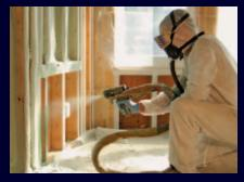
Insulation air barrier. Unlike fibrous insulation, properly installed spray polyurethane provides an excellent air barrier as it fills in around pipes, ducts, and wires and as it seals the gaps between framing and sheathing.
