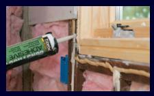
**Drywall air barrier.** Finished wallboard is mostly free of holes and can be made into an excellent air barrier by sealing around fixture boxes and along untaped seams. Caulk or adhesive on the framing prevents air movement.
