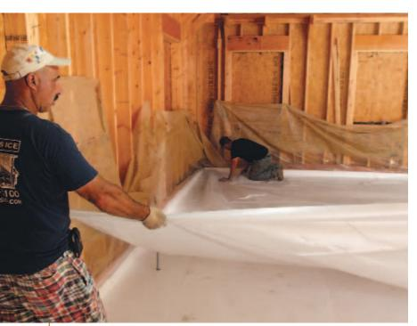
**Put poly under indoor slabs.** Soil contains more water than interior air. Without a polyethylene vapor barrier under the slab, moisture will move through the concrete and be released into the home's interior as water vapor. The plastic sheet should be installed above any subslab insulation.
