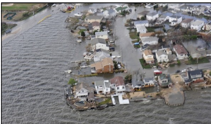
4-Foot storm surge hit many parts of Long Island southern coast
