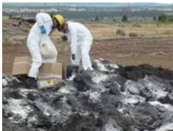
Figure 6. IXP ER ® 70C Calcium Peroxide being added to the soil treatment pile (July 2012)
