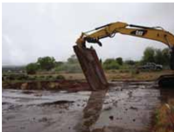
Figure 3. Breaking up concrete floor slab in former shop area to prepare for soil excavation (June 2012)
