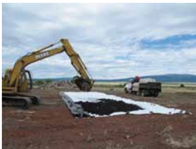
Figure 7. Construction of IXP ER 70C enhanced aerobic bioremediation soil treatment pile on liner (July 2012)
