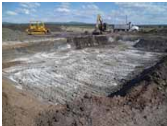
Figure 5. IXP ER ® 70C Calcium Peroxide placed in the bottom of the completed former shop area excavation (July 2012)
