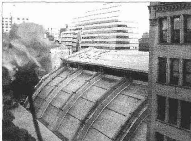
The roof of the Lexington Avenue armory. (Justin Rocket Silverman)
