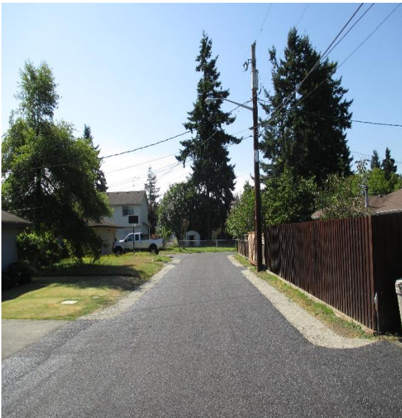
Porous Alley/ Wilson Av. ~ Puyallup, WA
