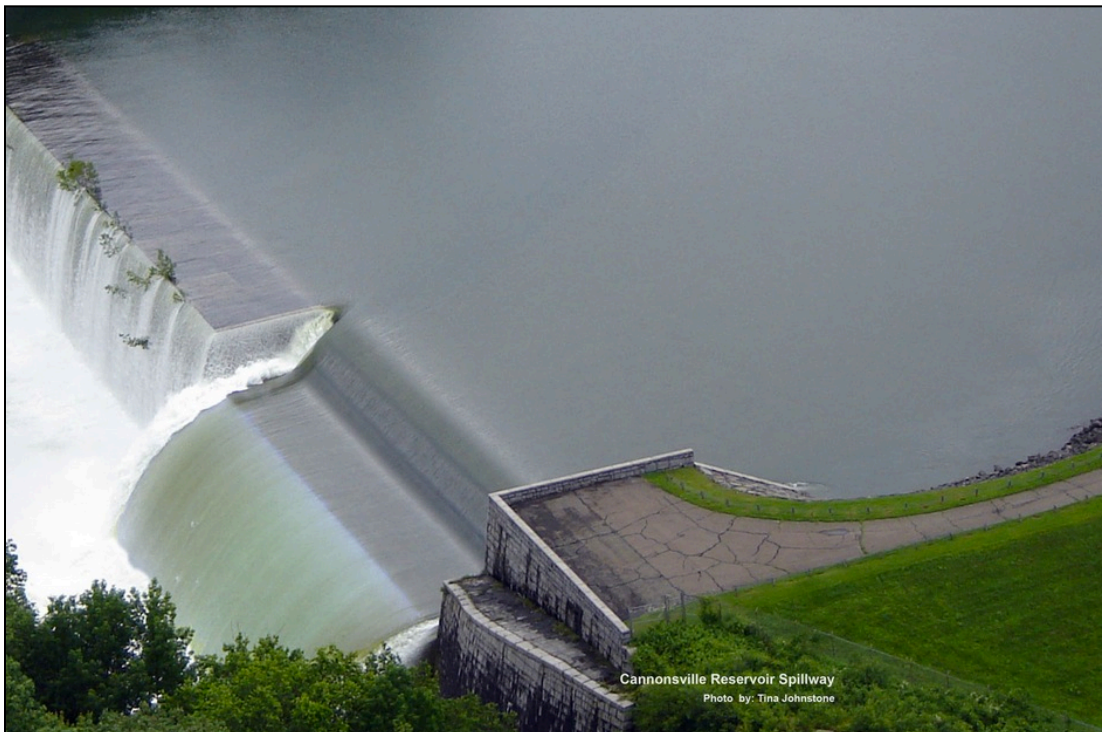
Cannonsville Reservoir Spillway
