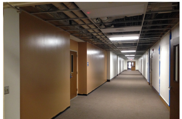
Phase 2 - Corridor Renovations
