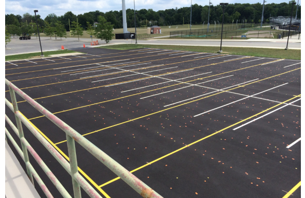
South Parking Area looking Southeast
