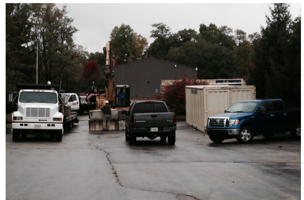
Temporary storage facilities during construction
