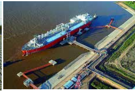
Completed work and operating dock
