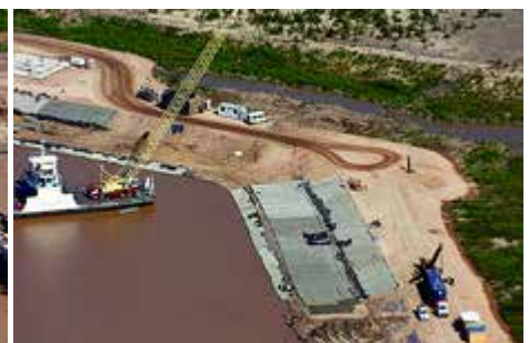
Installation of the precast blankets
