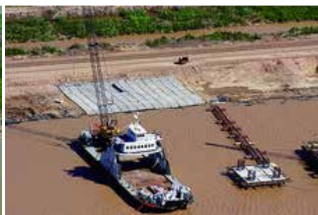
Precast blankets before installation
