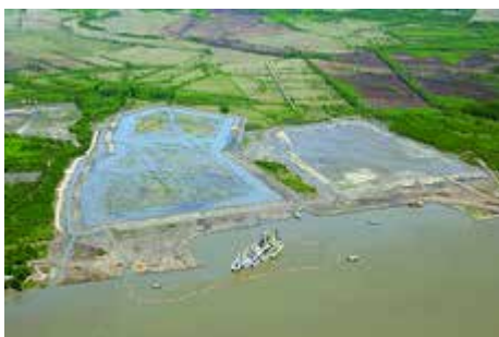
Dredging of the basin and filling the floodplain with dredge material
