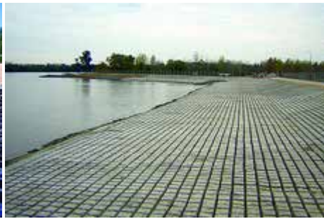
Coating of the berm and the superior slopes
