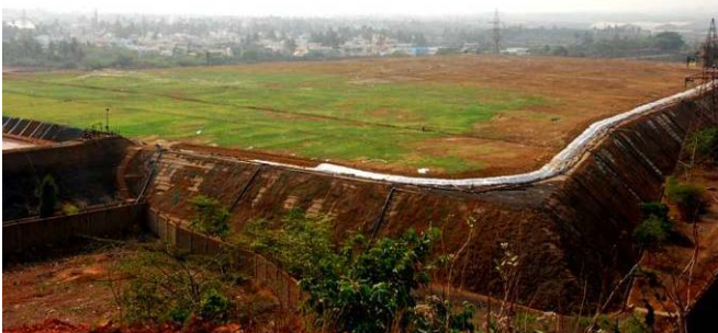
View of sludge pond after completion
