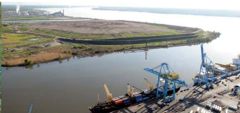
Completed berm looking across the Christina River
