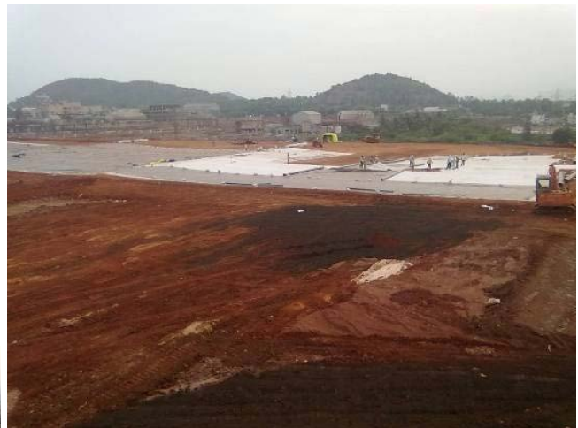
Construction of top liner system over geotextile stabilized layer
