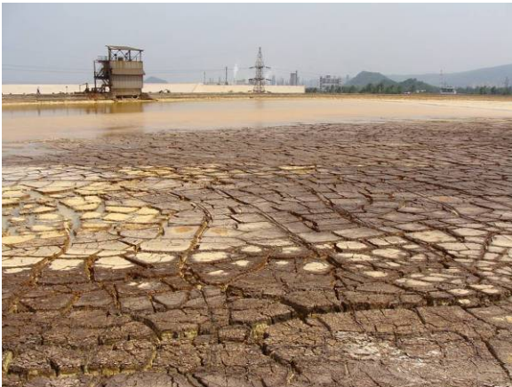
Sludge pond before closure
