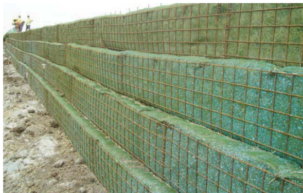
Berm facing using Miramesh®GR and wire basket forms
