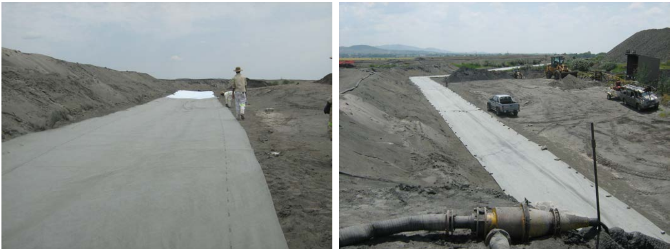
Kaytech supplies new drainage system to SamancorCr Tailings storage facility
