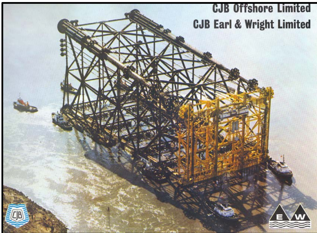
14,000 hp ocean tugboats move the Thistle Field Platform to the North Sea Oil Production Site
