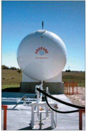
Since 2001, NFPA 58 has required safety upgrades of bulk storage tanks that are retroactive. The 2001 edition NFPA 58, section 2.3.3.2 (b) (2) c. Containers equipped with a positive shutoff valve that is located as close to the container as is practical in combination with an excess flow valve and retrofitted by July 1, 2011, with one of the following:
