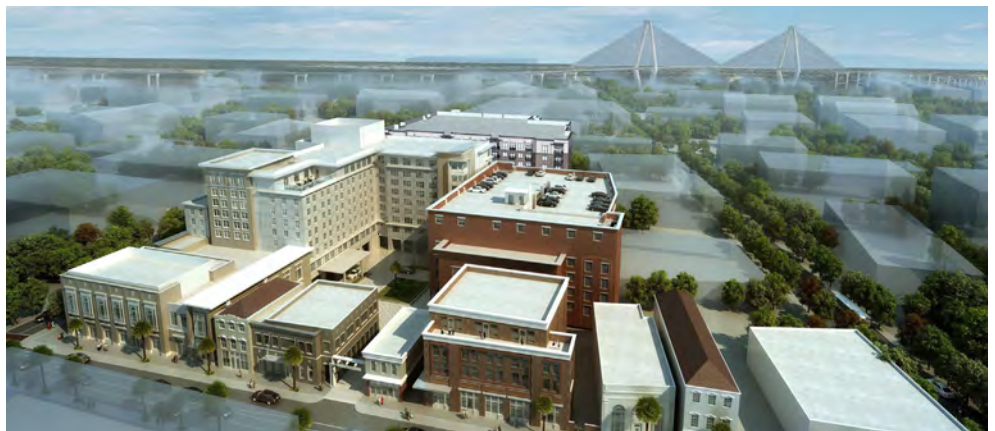
MIDTOWN - Regent Partners commenced construction on Midtown in 2013. The multi-use development will be the cornerstone of downtown Charleston’s Upper King Street and will feature over 16,000 SF of retail space.
