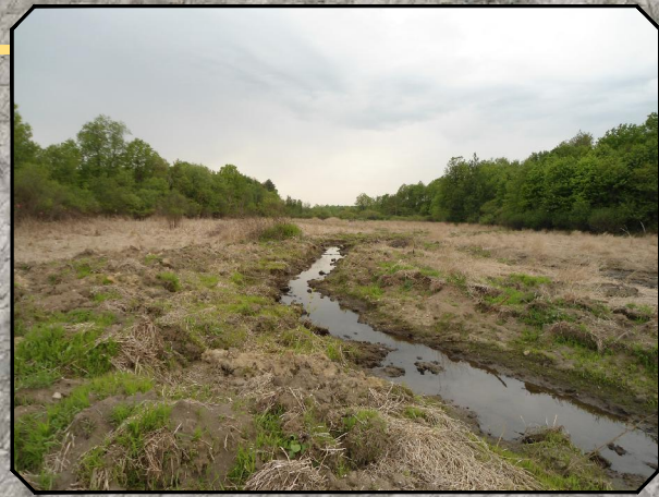
The previously straight ditch has been restored with meanders and is expected to develop morphological features more typical of other streams found in the Morgan Preserve (top left). The berms and the disrupted drain tile system have restored wetlands hydrology just several months after construction (top right).
